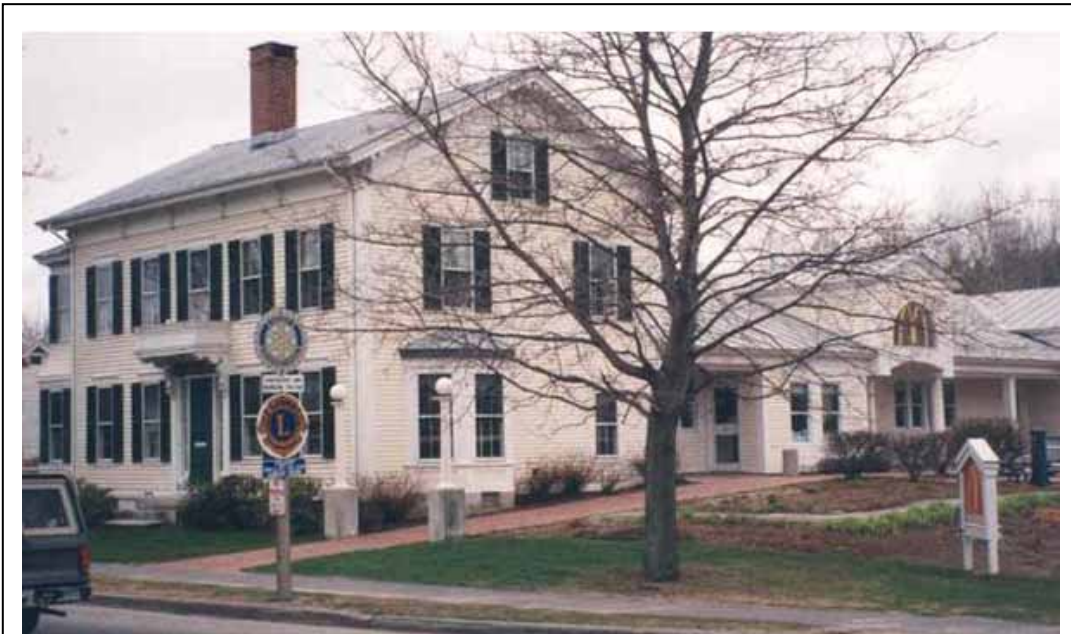
Figure 1—This fast food restaurant illustrates a significant departure from "off-the-shelf" standardized building design.
