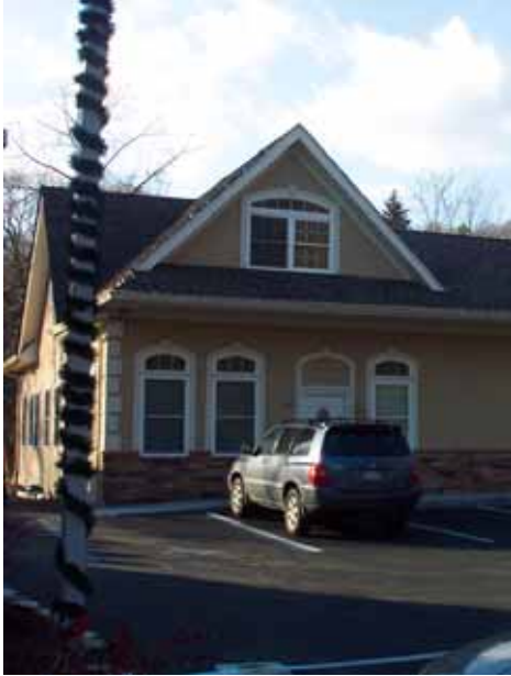
The peaked roof on this gas station reflects the built environment of Rosendale.
