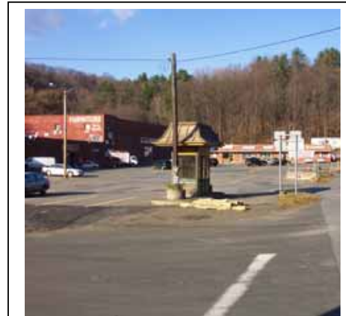
The former Fann's Plaza would benefit from improved landscaping and building designs that reflect Rosendale's character.
