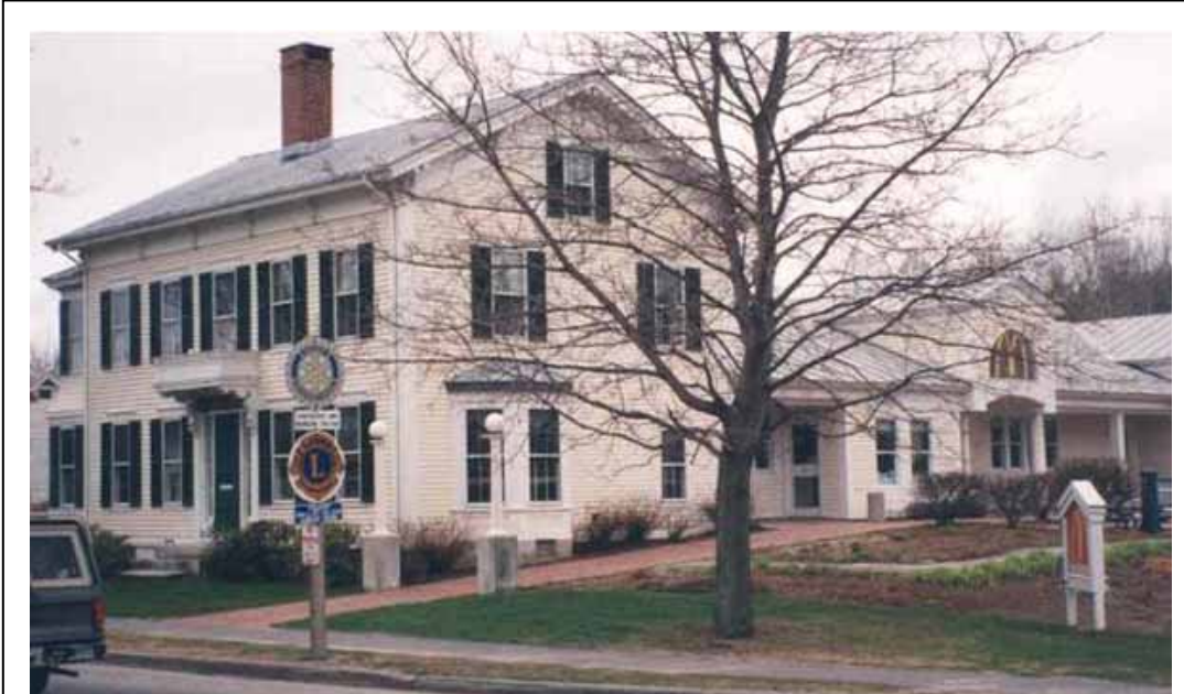
Figure 1—This fast food restaurant illustrates a significant departure from "off-the-shelf" standardized building design.
