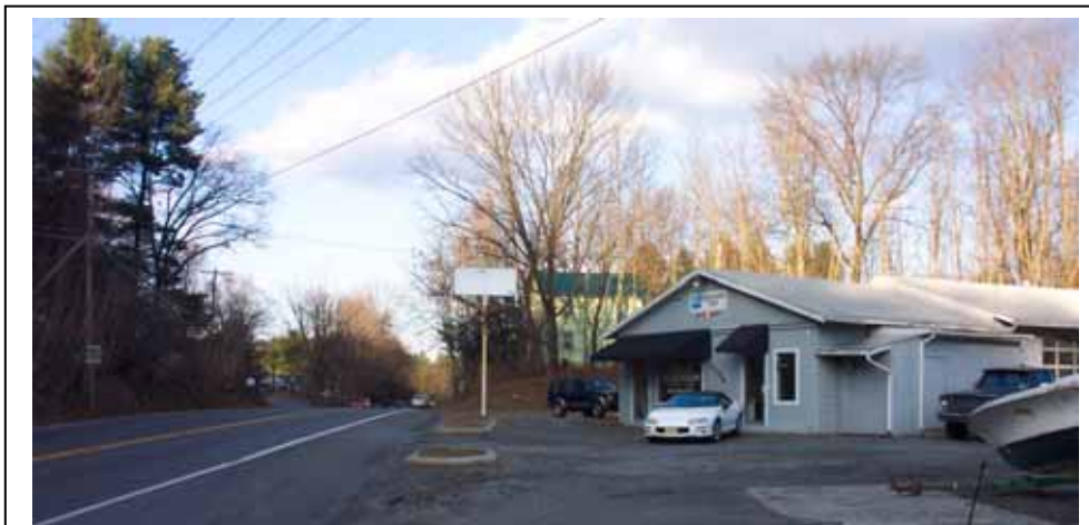
The two islands at this site suggest how even more landscaping would help separate the parking area from Route 32.
