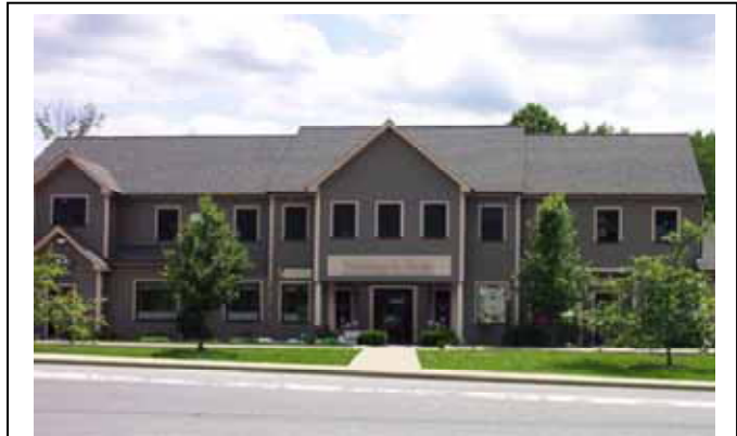
Figure 16— No wall that faces a street or connecting pedestrian walkway shall have a blank, uninterrupted length exceeding thirty (30) feet without including architectural features such as columns, ribs, pilasters or piers, changes in plane, changes in texture or masonry pattern, or an equivalent element that subdivides the wall into human scale proportions.
